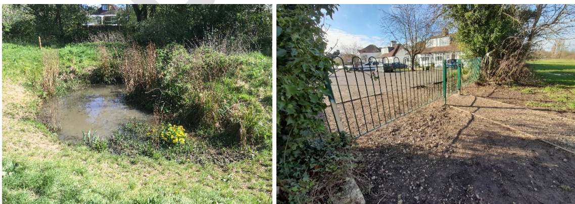
A selection of photographs showing interventions to improve flood resilience.
